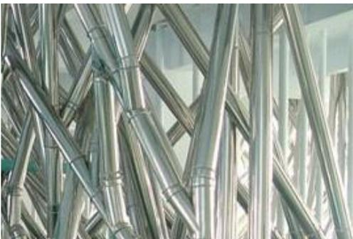
Gravity Spouting is used in a wide range of flour/feed and related material handling installations
